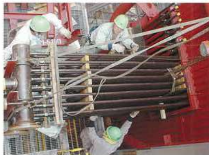
過熱器取込み Installation of super heater
