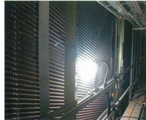
発電用ボイラ炉壁 自動溶射装置による現地溶射施工 On site spraying for the boiler tubes of the power station using the automatic spraying machine
