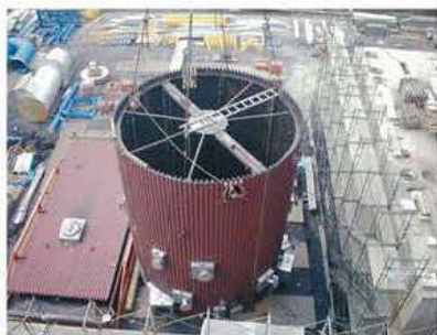
大型ガス燃焼室据付 Installation of large combustion chamber
