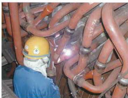
ステーブ連絡管 自動溶接 Automatic welding applied for connecting pipes for stave coolers
