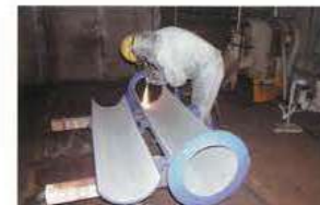
円筒内面の溶射施工 Wire spraying inside surface of the cylinder
