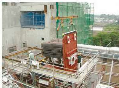
水冷パネル取込み(旗型管) Installation of a water cooled wall (Flag-shaped steam pipes)
